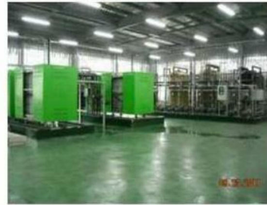
Clean water : 600 CMD Concentrate: 600 CMD EDR system
