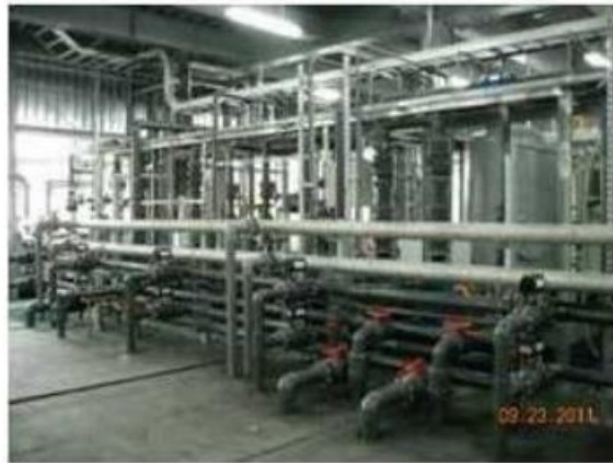
Flow rate: 1200 CMD Biological system (A 2 O/MBR)
